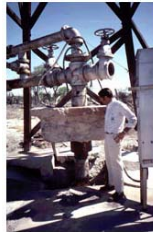
Figure 1. Photograph of Las Vegas Valley Water district Well No. 5 showing well-head protrusion caused by subsidence.
